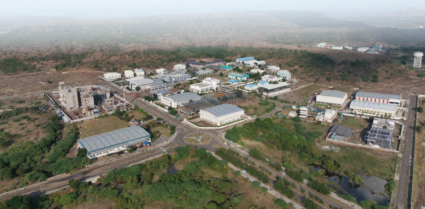
- Around Shendra Bidkin Industrial Area
